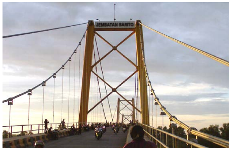
Figure 5. The Barito Bridge - http://www.google.co.id/
